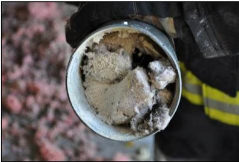
Clothes dryer venting systems can be a fire hazard if not properly installed and maintained. What happens? As clothes dry, moist air and lint accumulate inside the duct pipe, exterior exhaust vent and interior areas of the dryer.
